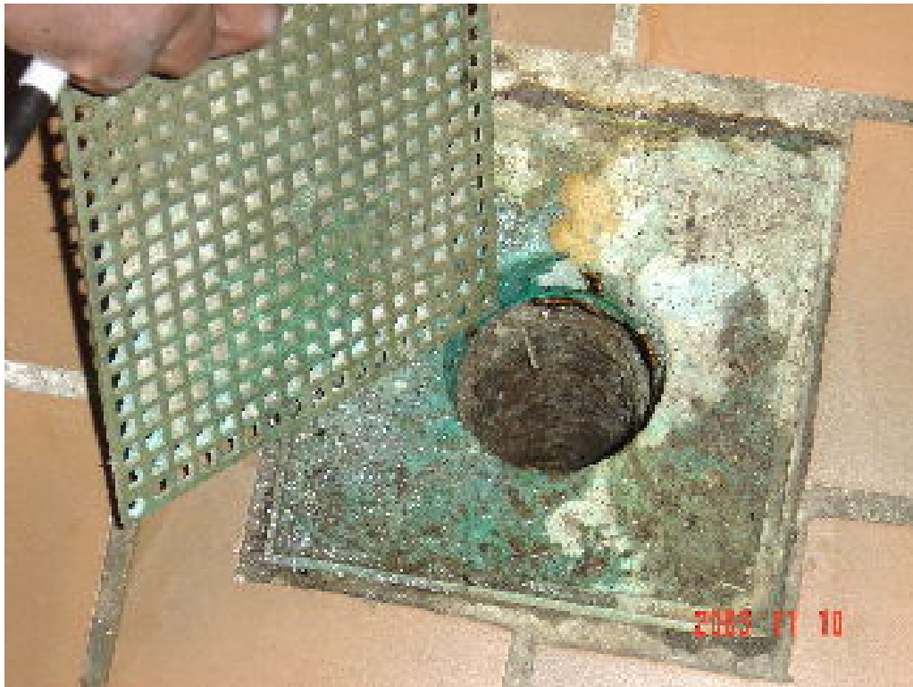
Clean floor drains and watch for cockroach activity
