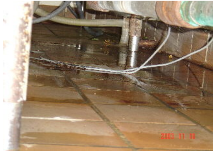
Report leaks to Facility Services in a timely manner
