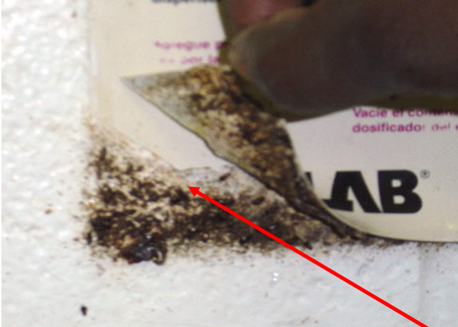
Watch for infestations of roaches in and around paper products such as posters and signs attached to walls and equipment
